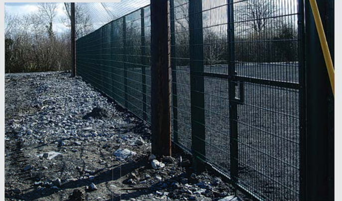
The Twin Wire system installed during the development of a site.
