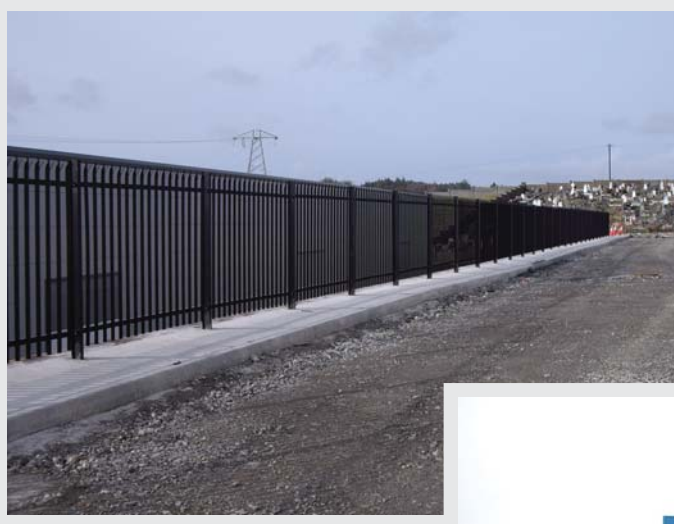
A newly installed palisade fence along a footpath
