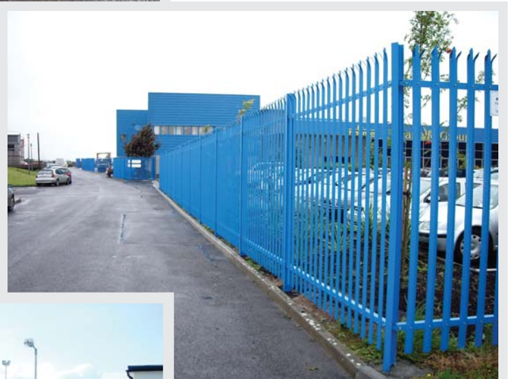
A matching powder coated palisade fence to suit the existing enclosed building
