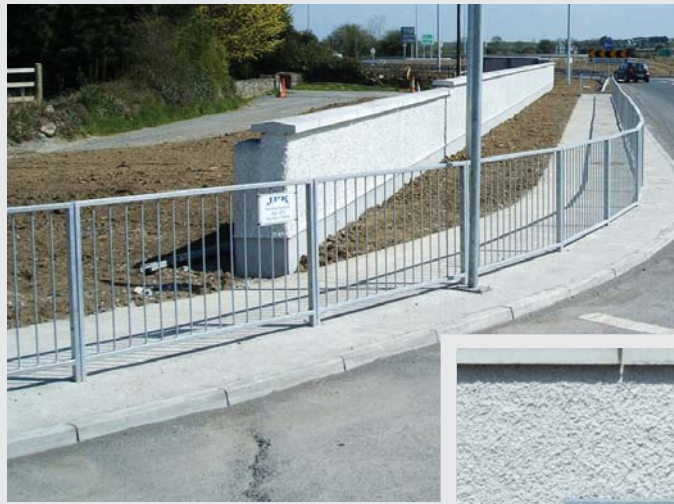
Pedestrian Guard Rail installed around a long curved footpath
