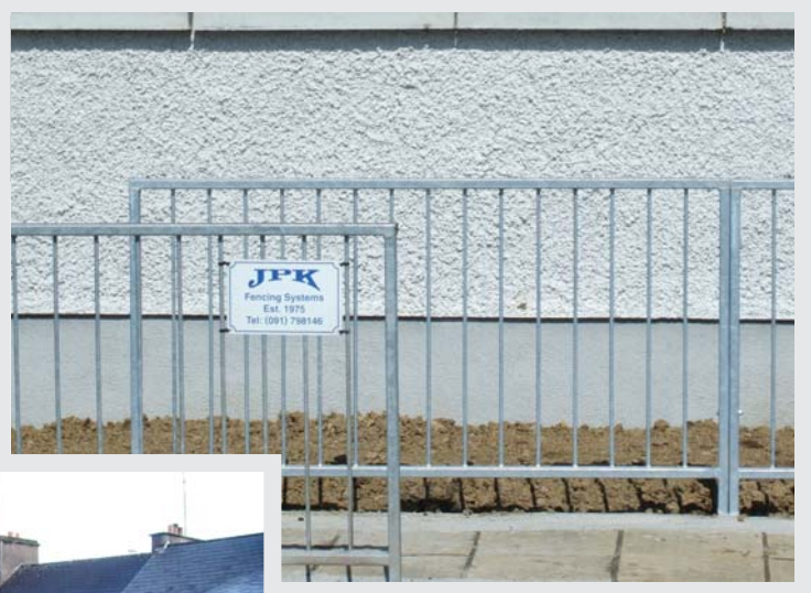
JPK installed Pedestrian Guard Rail to accommodate a pedestrian crossing
