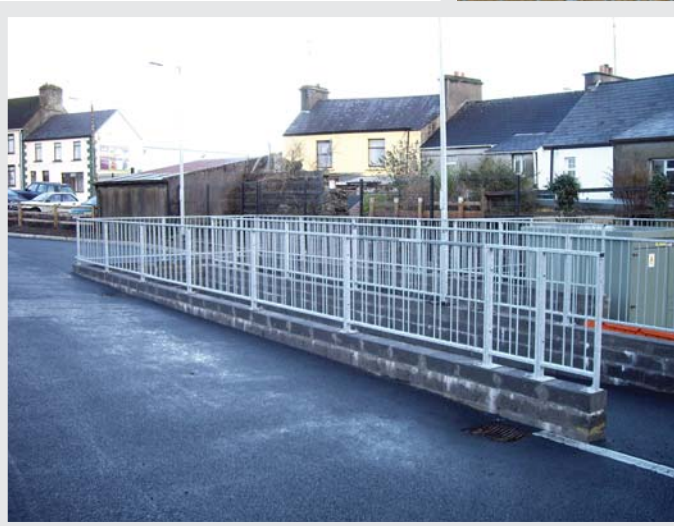
Pedestrian Guard Rail installed around a wheelchair access ramp
