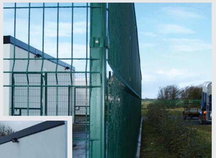
Close up of the corner assembly where the profile of the Alpha panel can be seen
